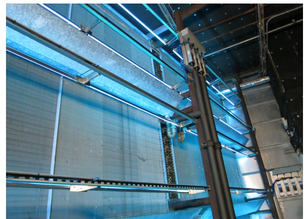
A large Fresh-Aire UV surface UVGI installation
