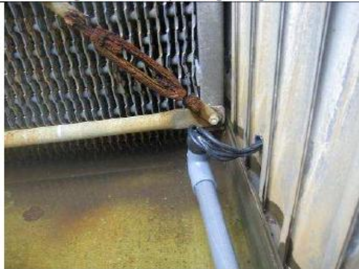
Figure C: Cable Penetration thru Wall of Cooling Tower
