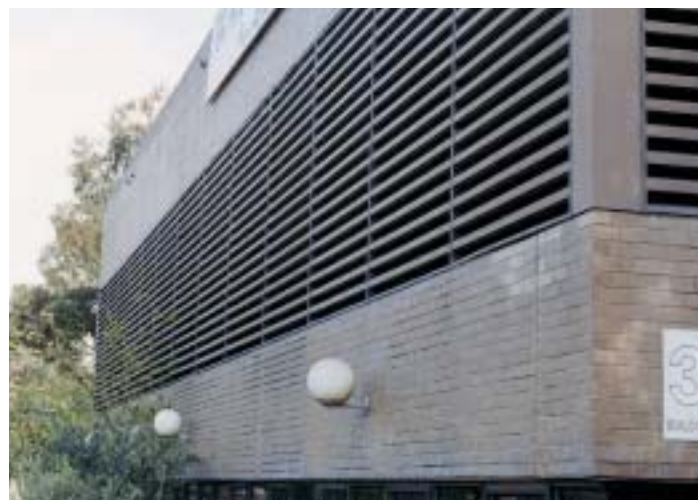
Multiple S-Line Louvre modules installed as a continuous wall
