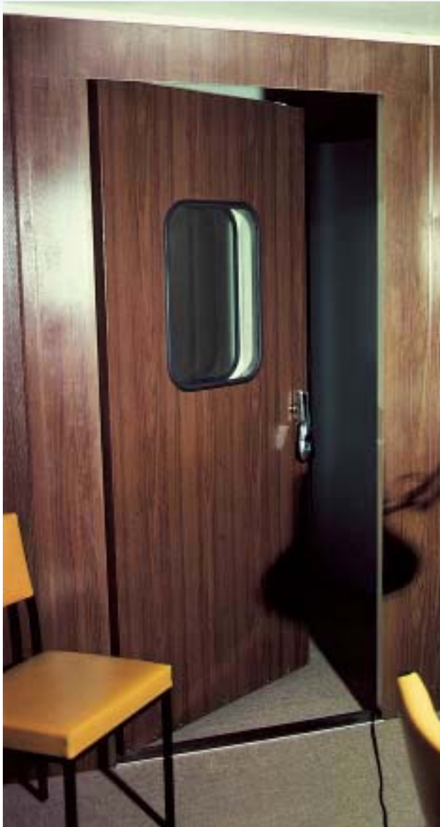
NAP Dyna door used at the entrances to the Audiology Testing Suite at the Lincoln Institute of Health Sciences, Melbourne.
