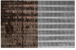
A biofilm on AC coils of only 0.002" can reduce efficiency by 37%! UV AHU Series 1 keeps AC coils clean and is the most costeffective and practical solution.
