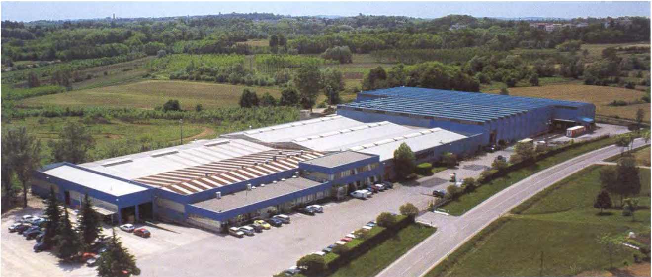
COMEFRI SpA factory at Magnano in Riviera (UD) – Italy with 14.500 m 2 workshop. Production of radial fans for airconditioning and general ventilation.
