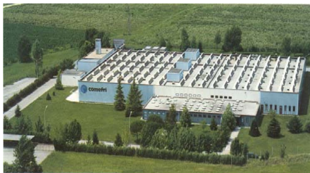
COMEFRI SpA factory at Artegna (UD) – Italy with 6.300 m 2 workshop. Production of industrial fans and special executions.
