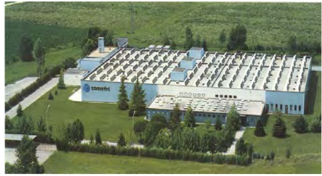
COMEFRI SpA factory at Artegna (UD) – Italy with 6.300 m 2 workshop. Production of industrial fans and special executions. Test facilities: laboratory accredited by AMCA and SINAL.
